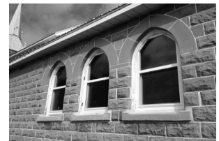
New windows at St Barnaby's
