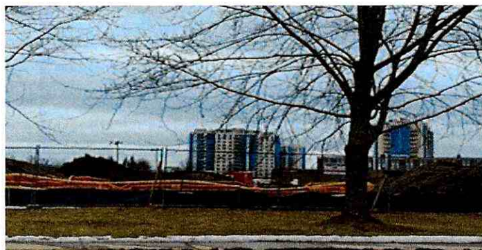
Construction is underway on the new Kingston East Community Centre.
